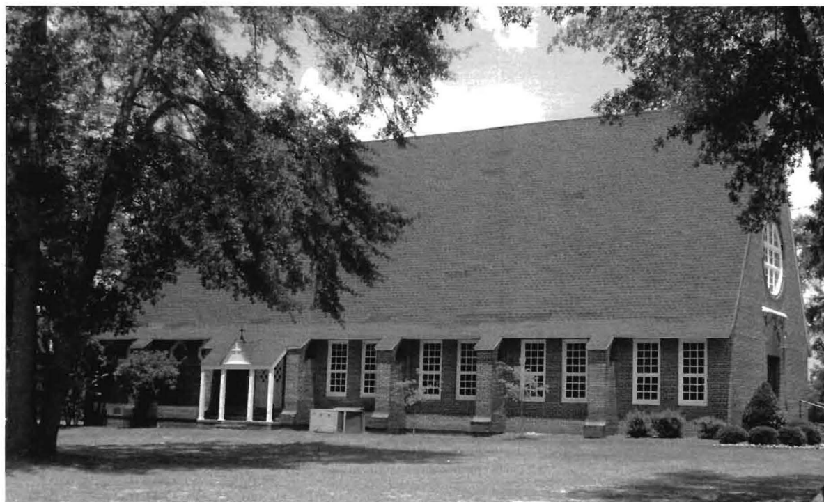
FIGURE 15 (BELOW) S. J. Makielski, St. Philips Chapel, Voorhees College, Denmark, South Carolina, 1936, side elevation. (Photograph by author)
