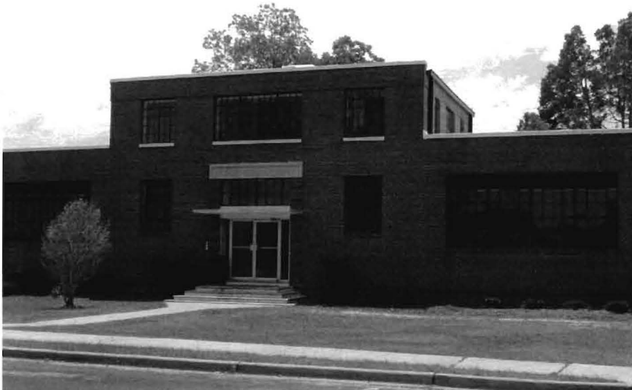
FIGURE 13 S. J. Makielski, St. James Building, Voorhees College, Denmark, South Carolina, 1932 front elevation. (Photograph by author)
